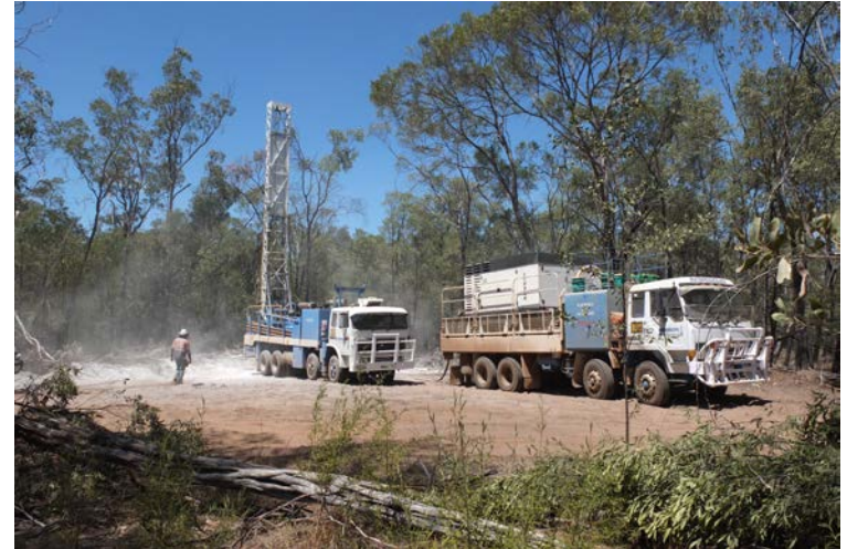
Drilling ML20 at West Bowen's "Moorlands Deposit" in October 2012
