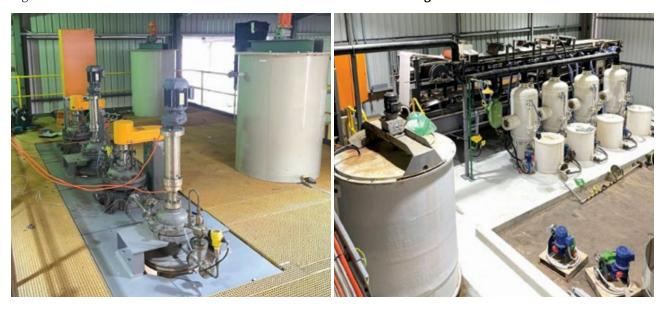
Figure 4 – Demonstration Plant. Left: Iron oxidation and precipitation circuit. Right: Installation of iron polishing and MHP precipitation circuits.
