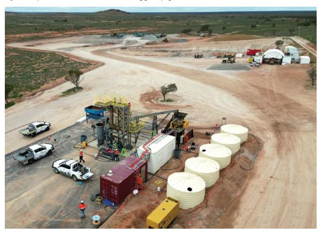
Figure 8 – Multi-stage crushing plant processing ore stockpile in preparation for milling.
