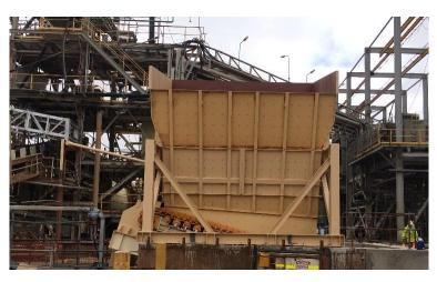
Photo 5: New Mill 1 feed hopper installed
