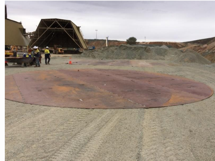
Photo9: New leach tank floor
