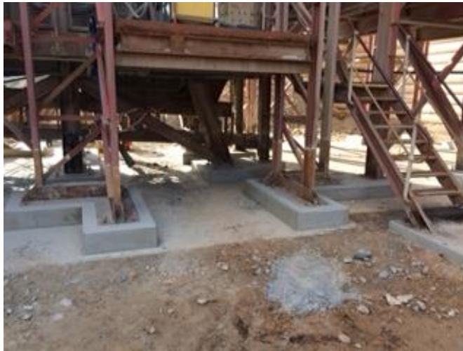
Photo2: Repaired Crusher Footings
