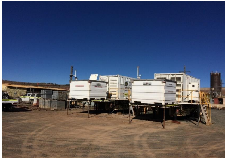
Photo10: Diesel generators installed
