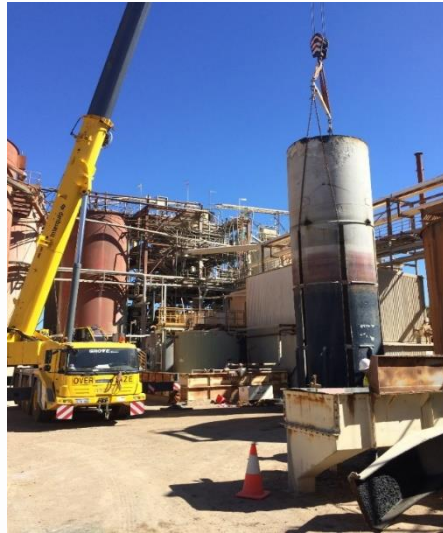
Photo8: Final Leach Draught Tube Removed
