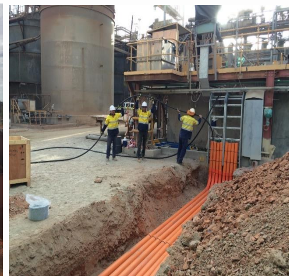
Photo6: Running cable to Mill2
