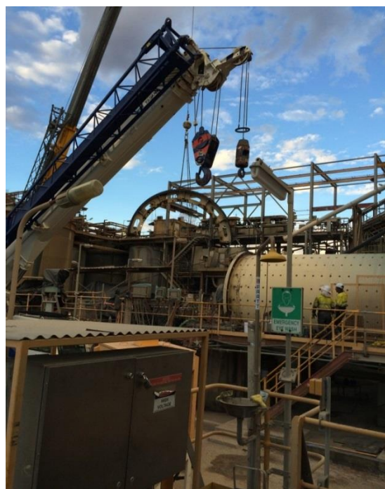
Photo 3: Removal of Mill 2 Girth Gear
