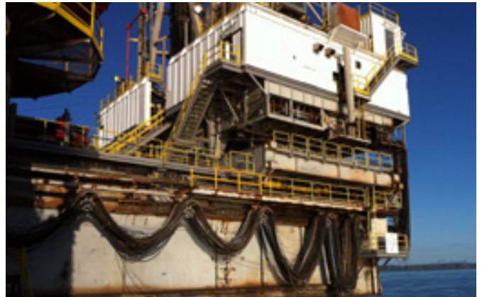
DRILLING PLATFORM CANTILEVERED OVER COSMO 1 PROSPECT
