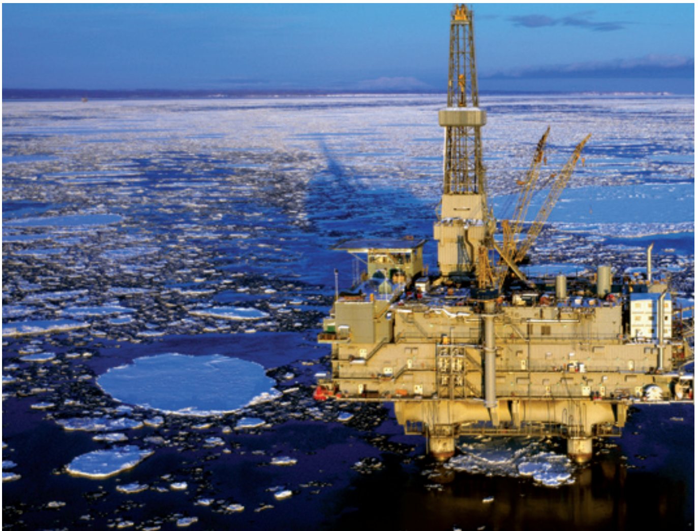
NORTH COOK INLET UNIT EXISTING TYONEK PLATFORM
