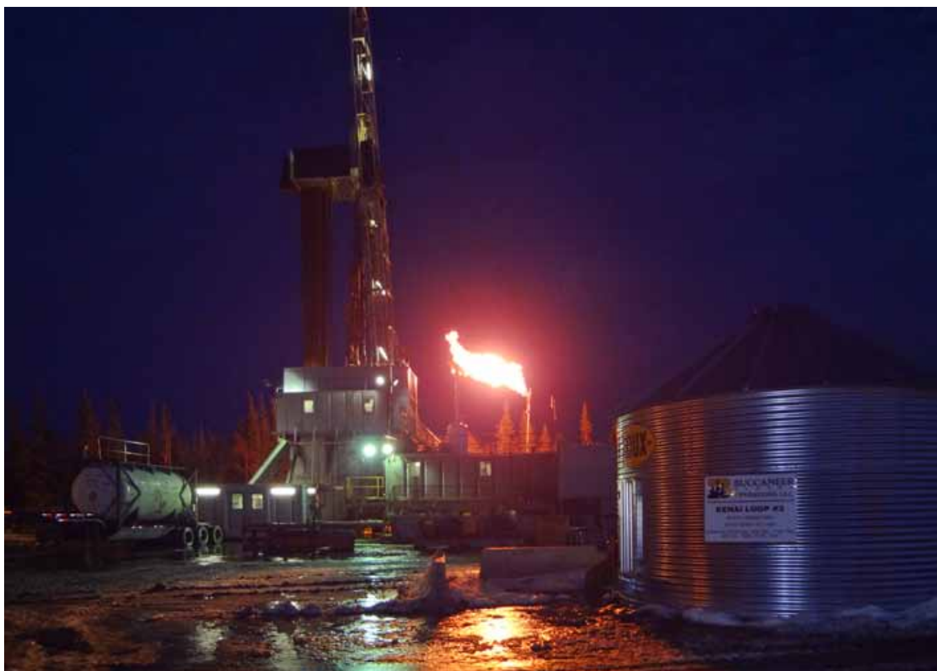
KENAI LOOP #4 GAS FLARE
