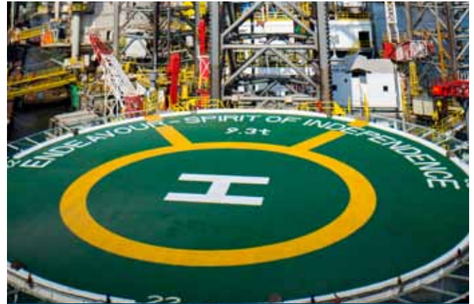
CLOSED UP VIEW OF THE HELI DECK. SOME PARTS HAVE BEEN PAINTED BY KFELS
