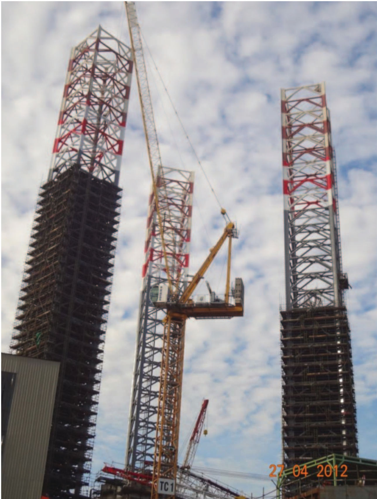
LEGS AFTER PAINTING- DE-STAGING IN PROGRESS
