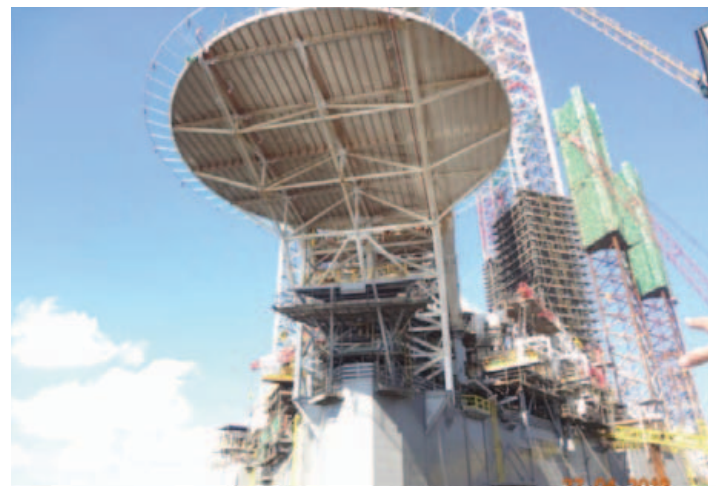
UNDERNEATH VIEW OF THE HELIDeck
