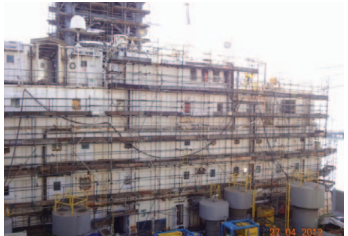
LIVING QUARTER VIEWED FROM THE PIPES STORAGE DECK
