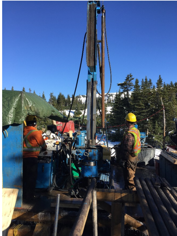
Drilling operation at Panorama North
