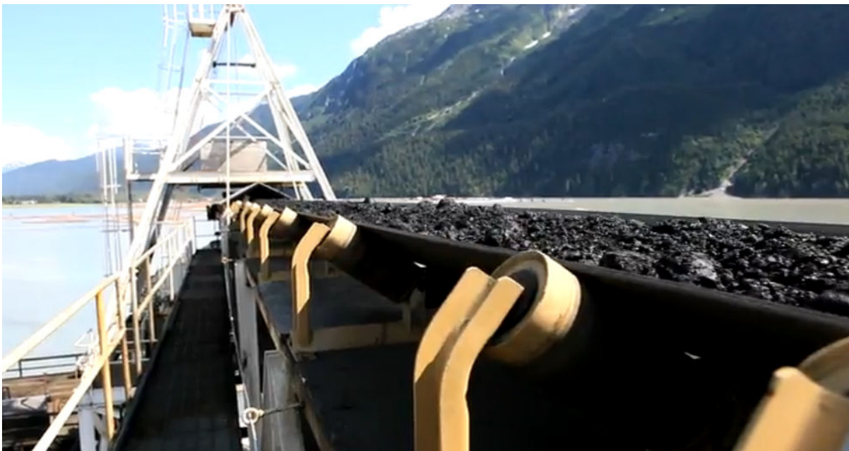
Testing the ship-loader conveyor
