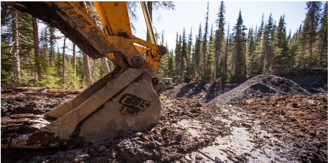
Excavation of S80 outcrop at Groundhog North
