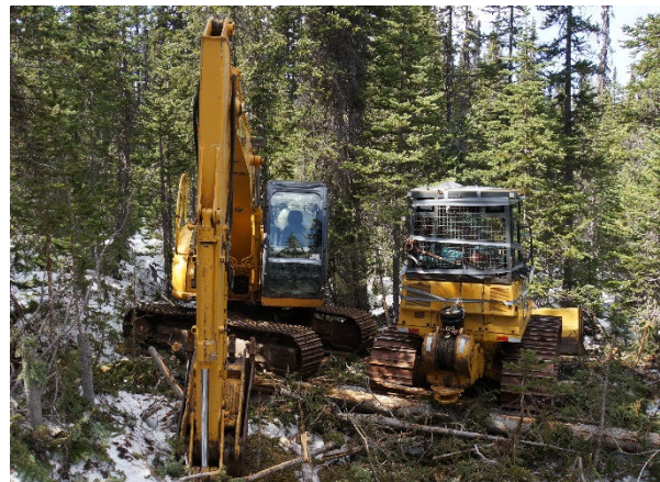
Trenching and portal development machinery
