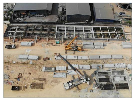
Figure 4 – OSD Tank Roof Panel Fabrication
