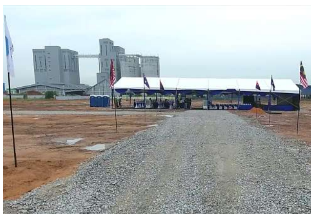
HPA plant site – Tanjung Langsat, Malaysia
