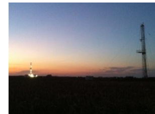
Two Rigs Drilling Verticals Dan Darling Drilling
