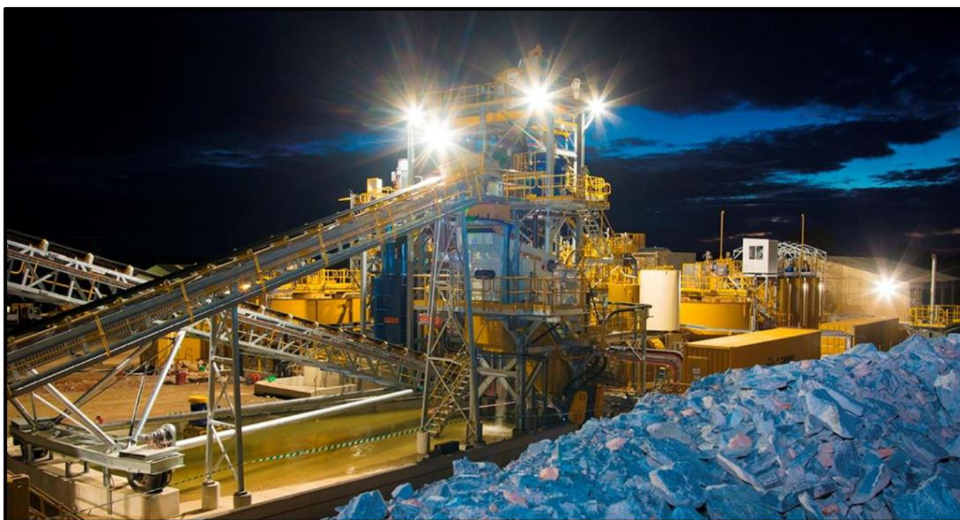
Hera Processing Plant
