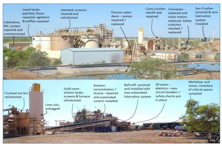
Figure 3. Coyote Gold Plant refurbishment nearing completion. Top image is view to southeast and bottom image is view to northwest
