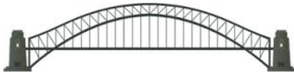
Sydney Harbour Bridge for scale
