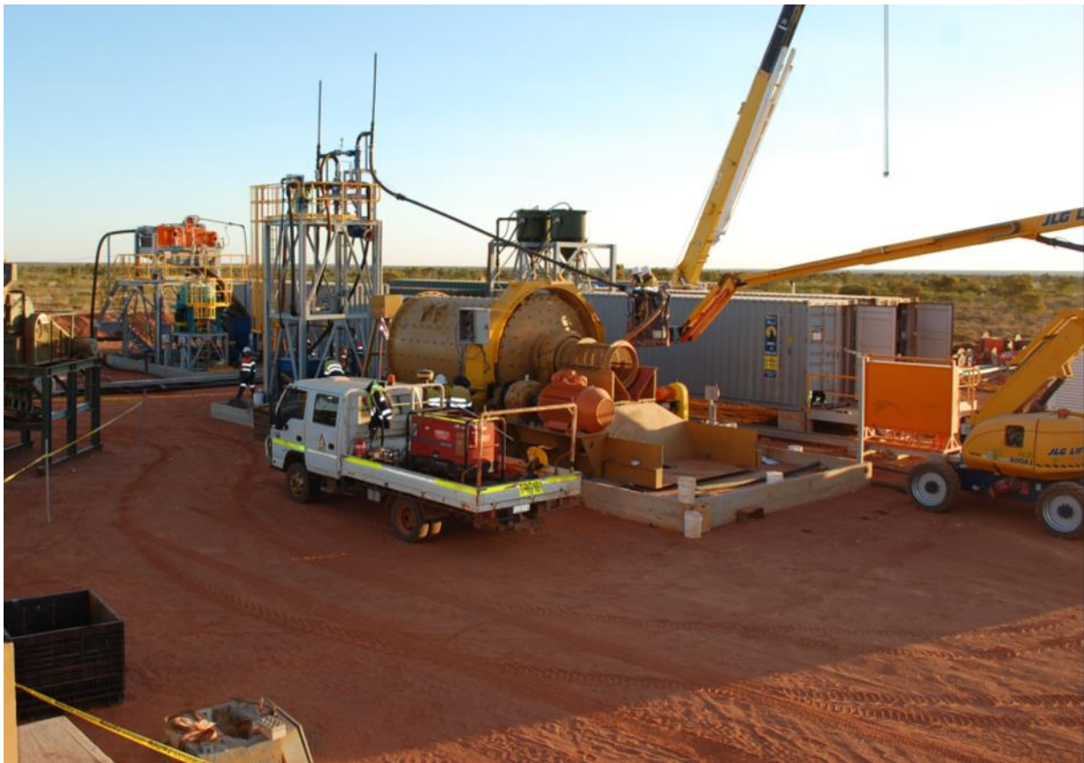
Figure 3. View from atop the crusher of ball mill and Knelson concentrator.
