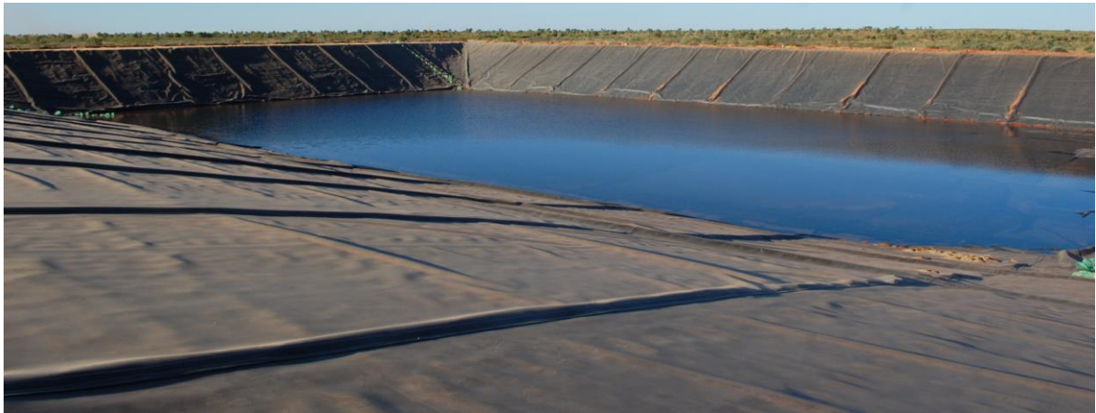
Figure 5. Lined tailings / process water storage facility and being filled with water for processing.
