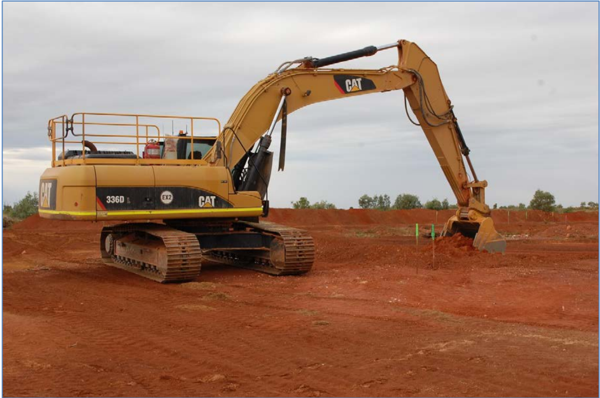
Figure 3. First digging at the Golden Hind.
