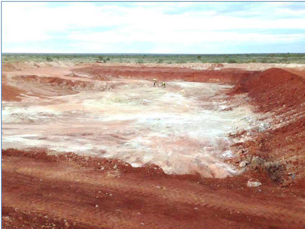
Figure 2. Photograph of Tailings Storage Facility.
