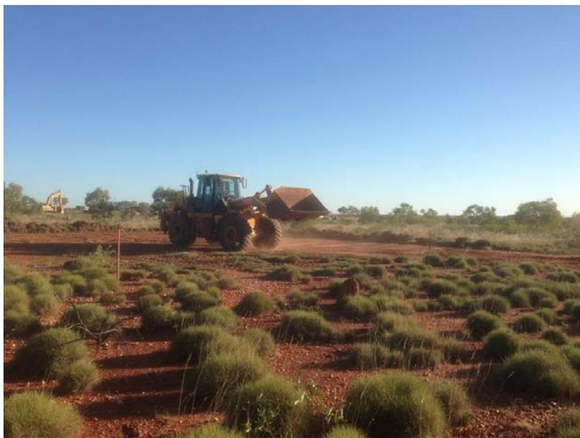
**Photograph 2. Clearing of topsoil at the Pilot Plant location**
