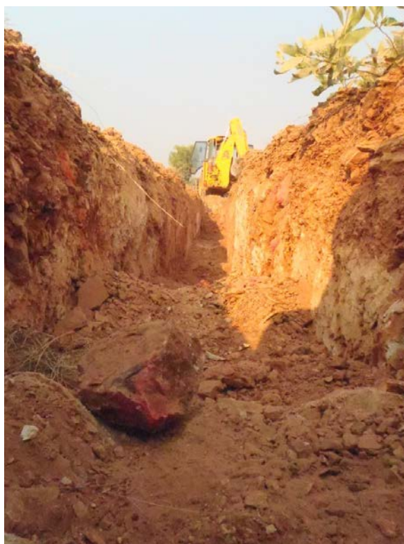
Figure 3. Backhoe operating within one of the trenches at Old Pirate.
