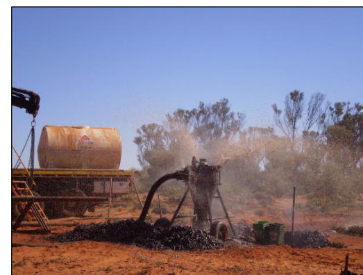
Piercing the clay lithologies into the basal sand aquifer produces high-pressure, hyper- saline brine flows
