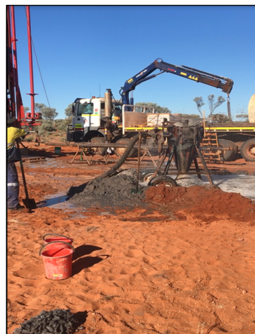
Figures 5 & 6: Right, piercing the basal sand layer and channeling the natural overflow to containment bund
