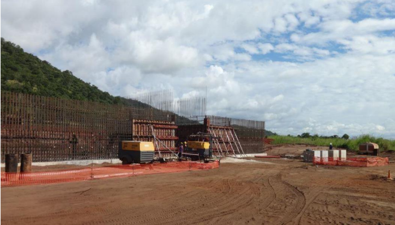
Figure 4 – Balama crushing facility foundations
