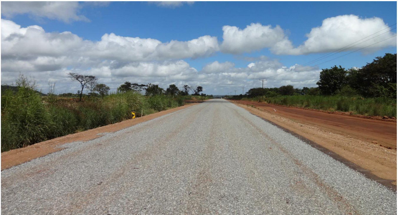
Figure 6 – Preparation of the access road surface for bitumising
