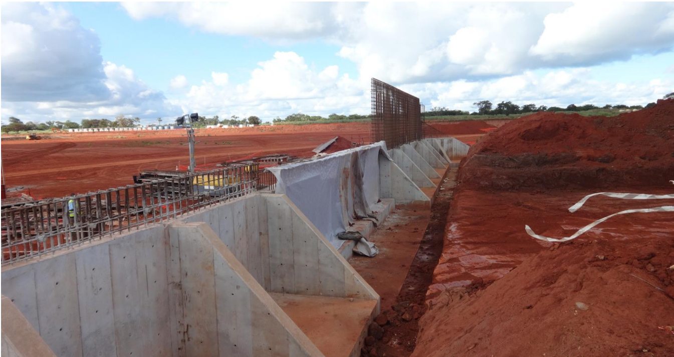
Figure 5 – Balama ore bin back wall
