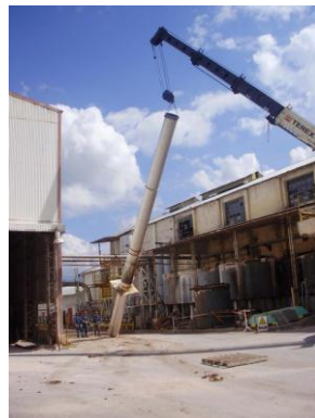
Boiler stacks being removed and loaded for relocation
