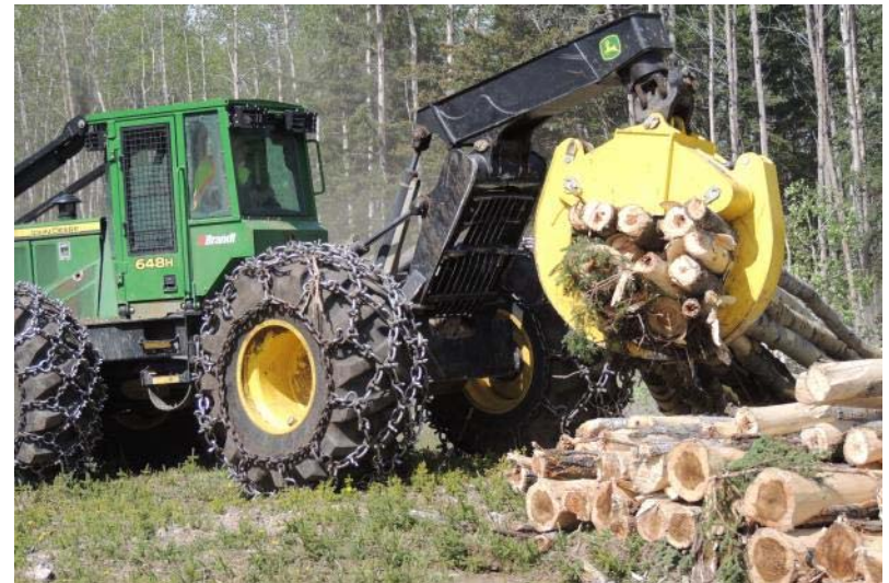
Coalspur (Alberta, Canada) 6.5km rail siding clearing (2013)
