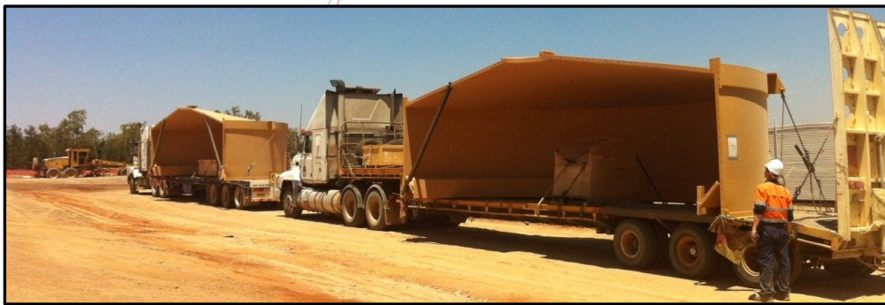
Leach feed thickener tank arriving on site
