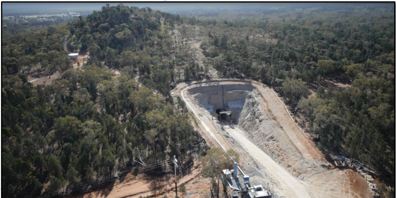
Hera Boxcut and Portal
