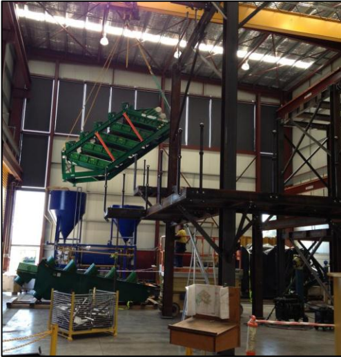
Derrick Screen being fitted to top frame
