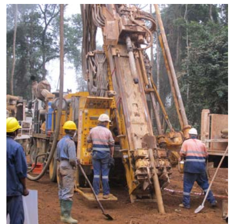
Figure 3: Wallis rig in action at Makengui
