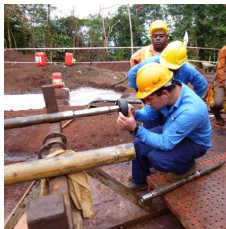
Figure 2: Orientating drill bit
