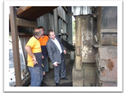
Coldry Business Manager Ashley Moore (right) inspecting the test with BAIC personnel
