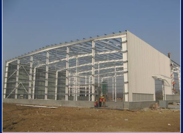
Lithium Packaging Building Steelwork
