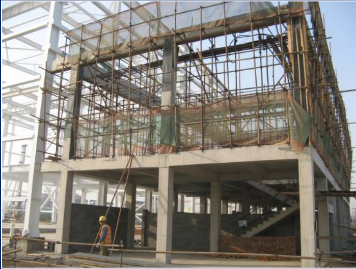
Admin and Maintenance Building
