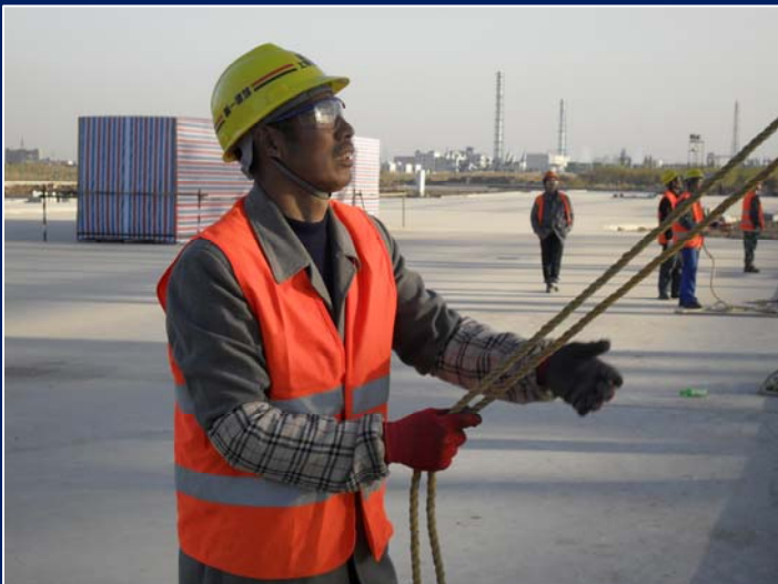
Safety focus on site
