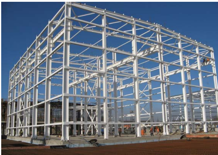
Maintenance Workshop Steelwork
