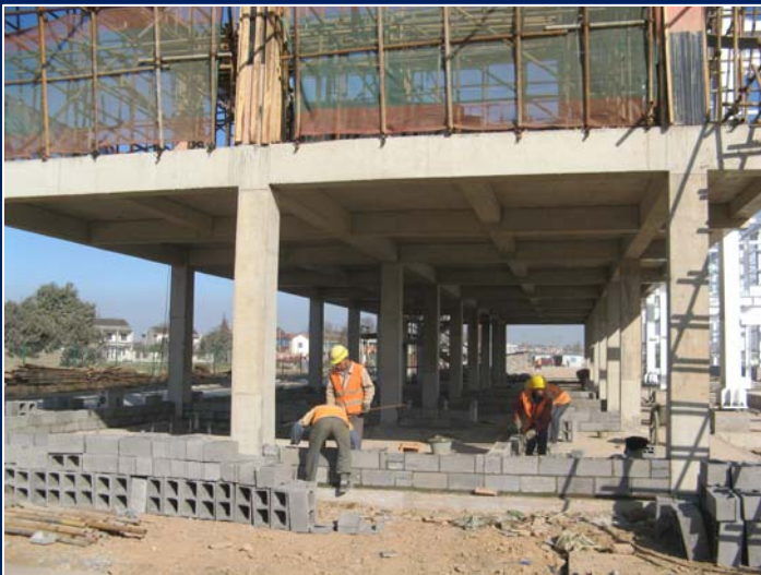
Brickwork of process building
