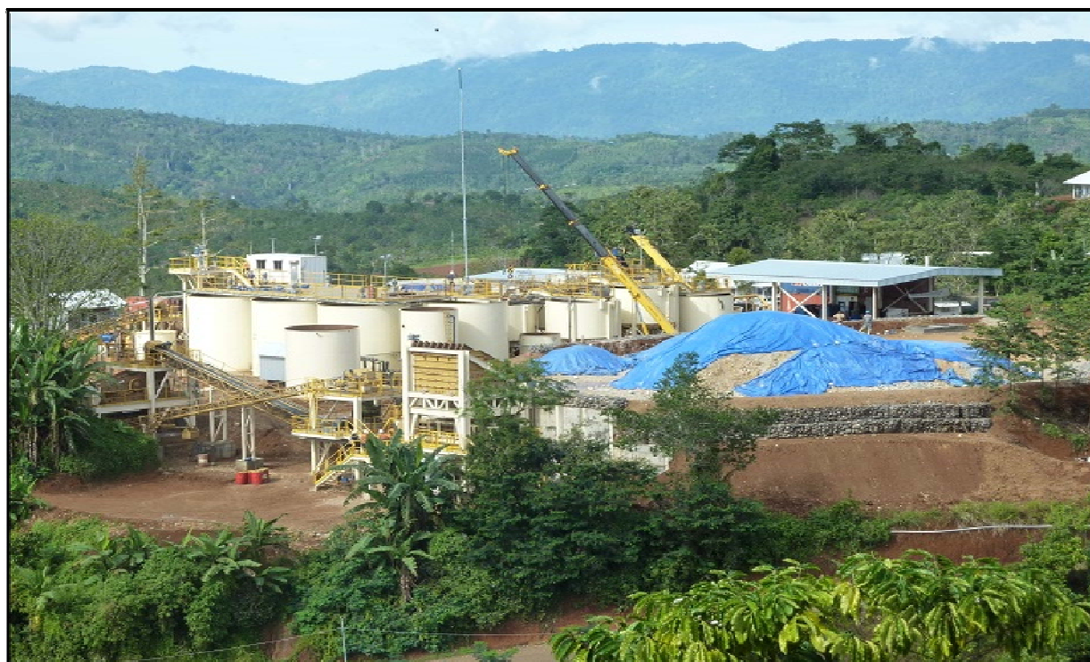
Figure 1. Way Linggo processing plant during commissioning with high grade ore on the crusher ROM pad
