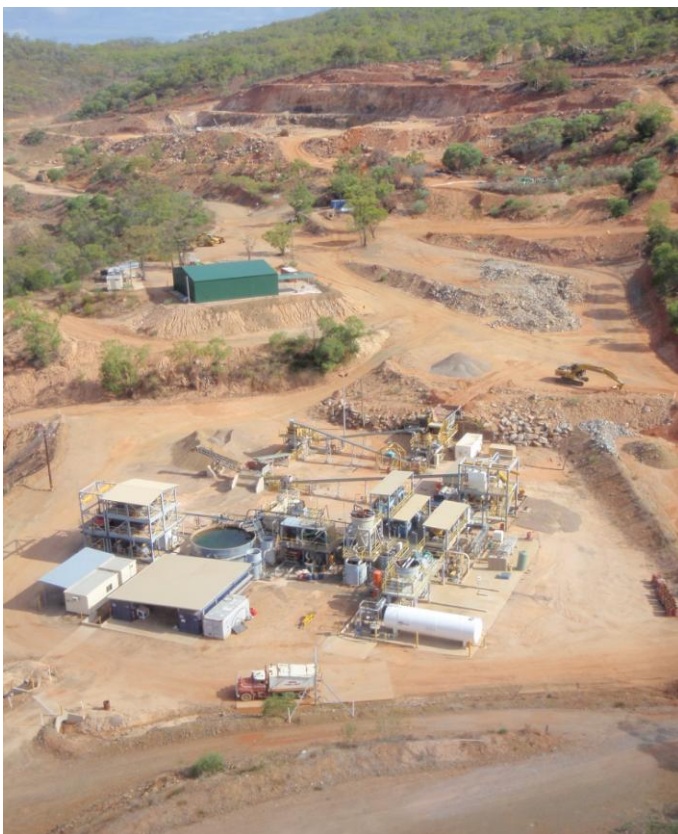
Wolfram Camp's existing 150,000tpa processing plant
