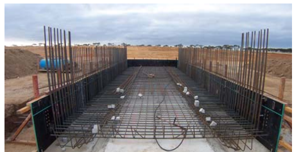
Formwork on Site
