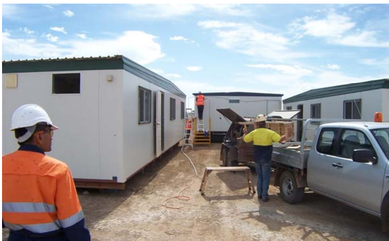
Site construction office
