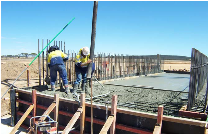
Concrete works at fine ore bin
