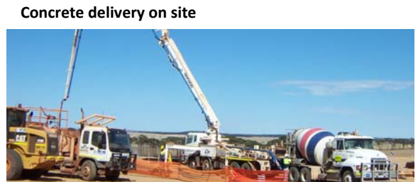
Concrete delivery on site
