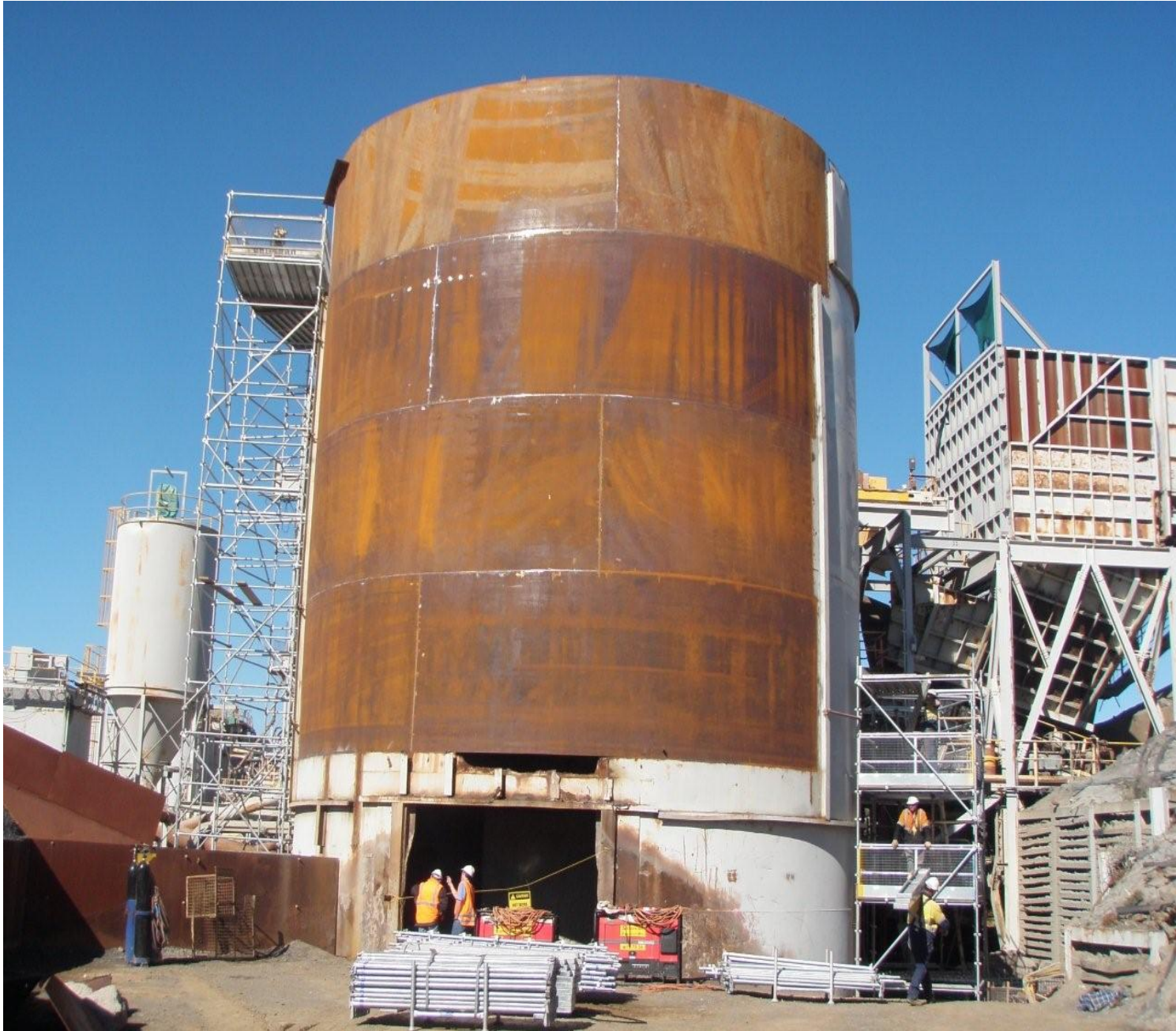
Figure 8: Rebuilding the fine ore bin
