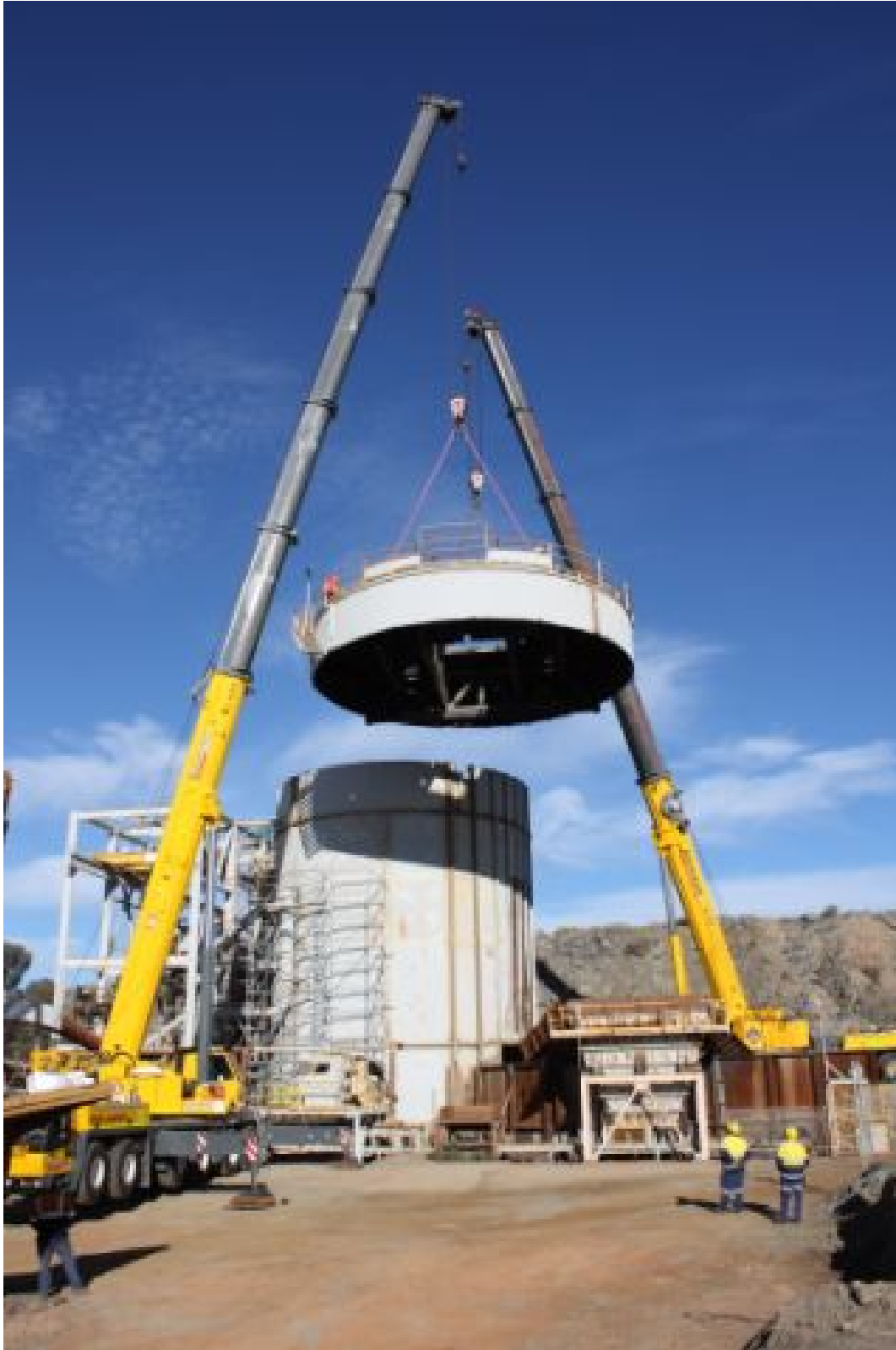
Figure 7: Dismantling fine ore bin for refurbishment
