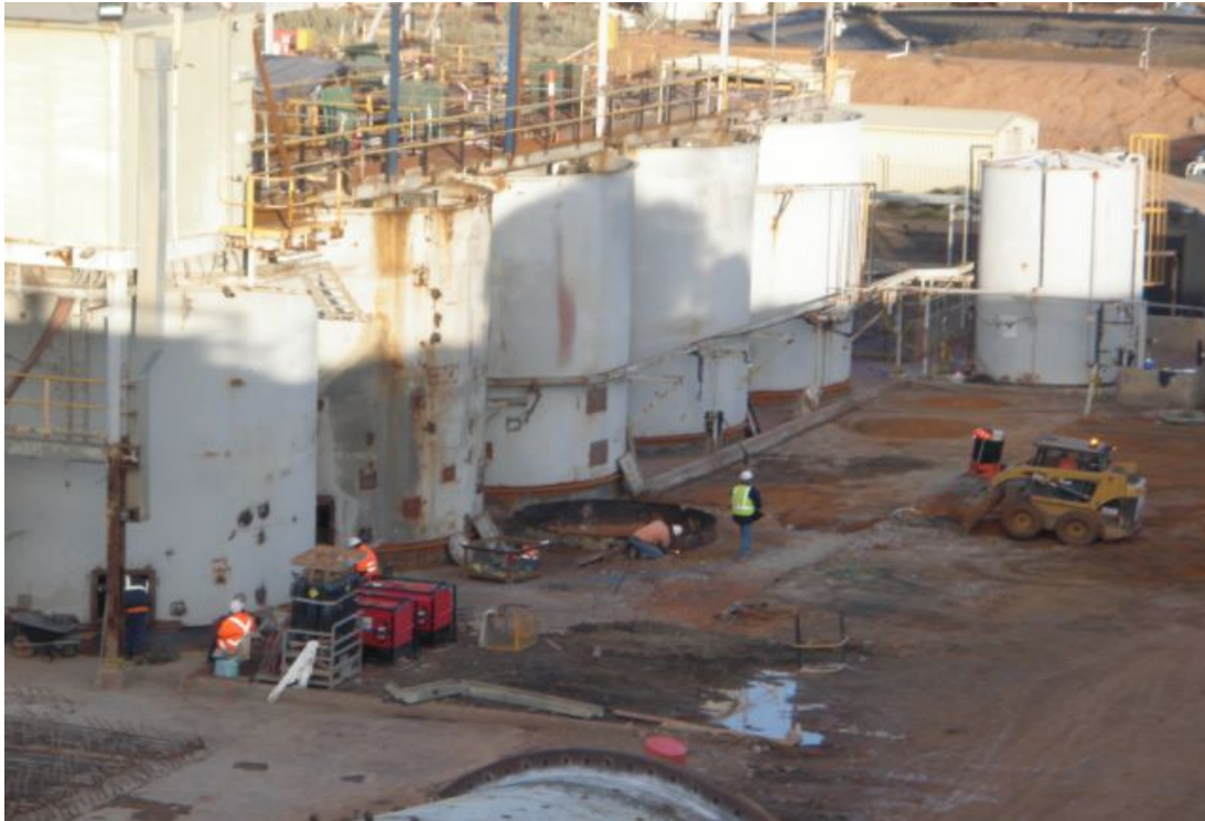
Figure 12: Refurbishment of CIL tanks and infrastructure
