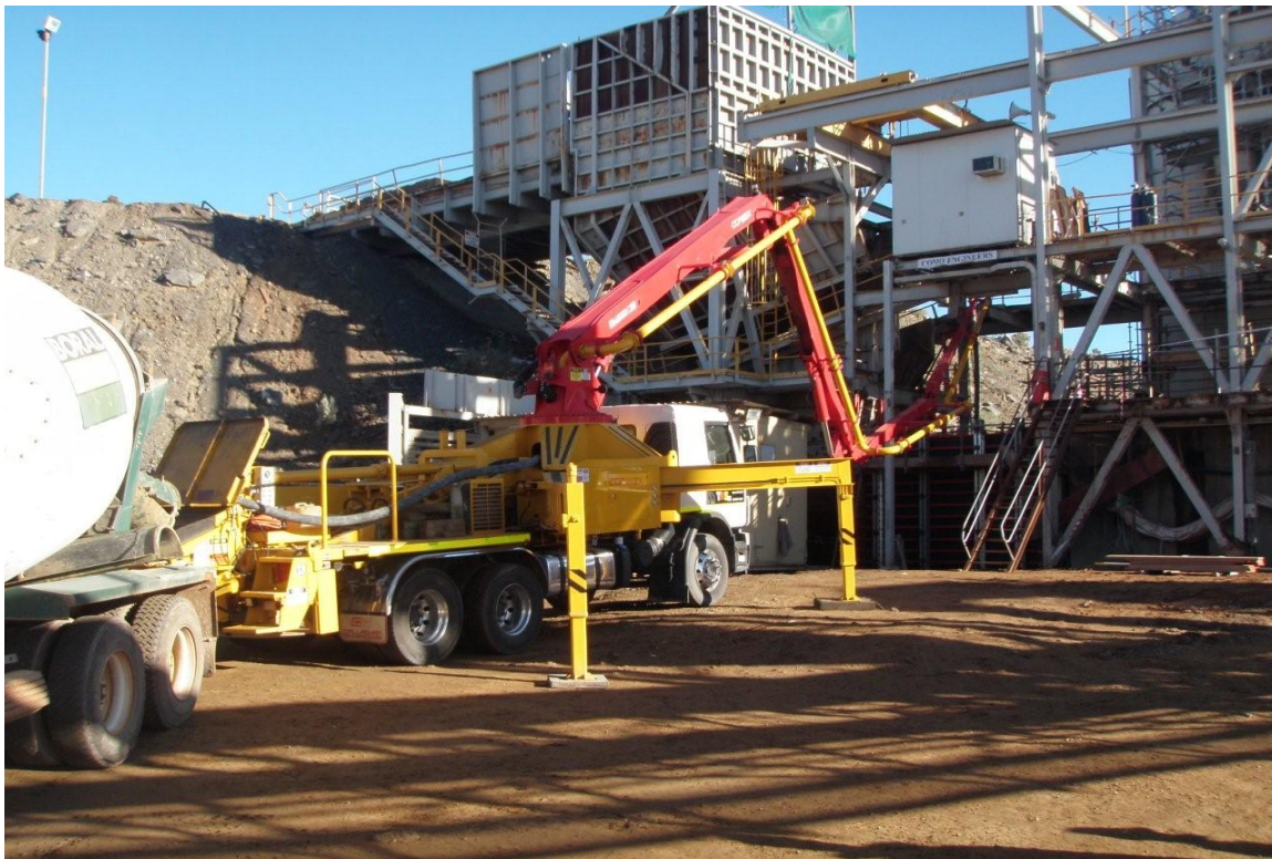
Figure 5: Pouring Concrete for Primary Crusher Foundations
