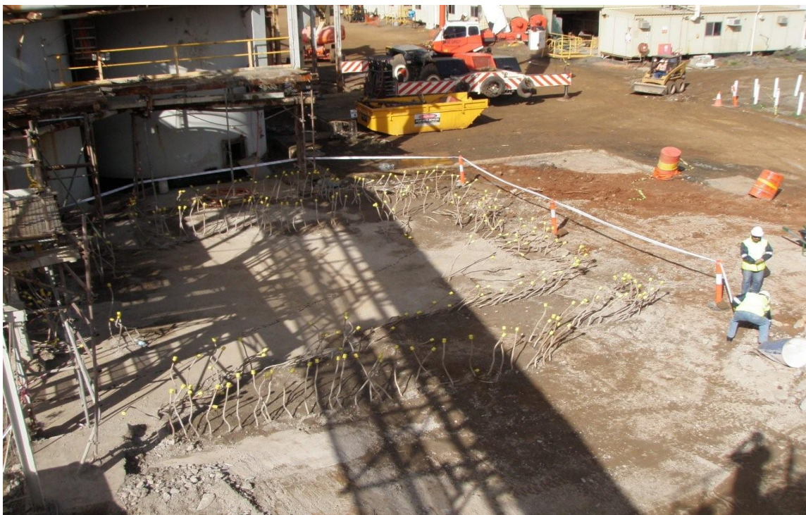
Figure 10: Foundations ready for new concrete
