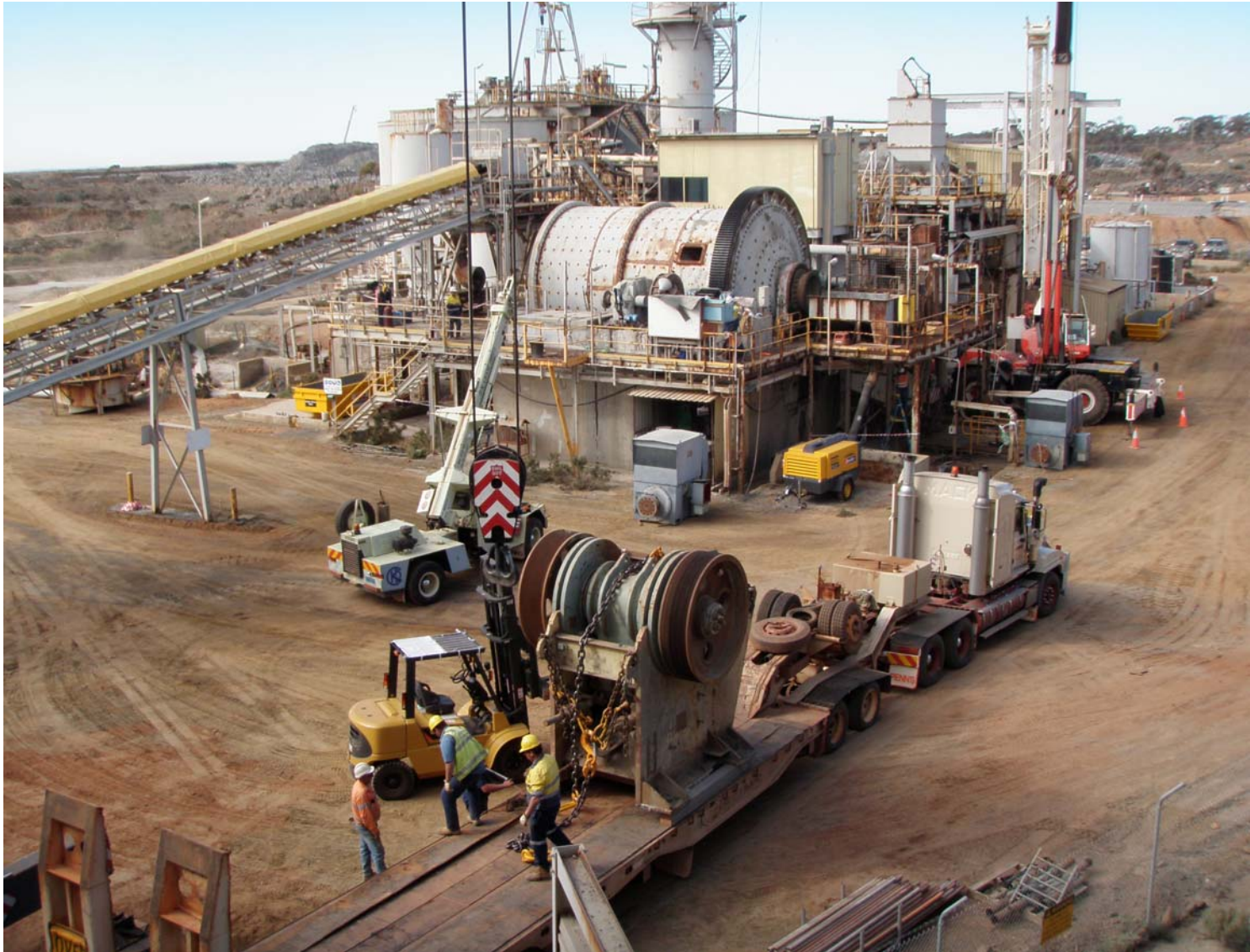
Figure 3: Primary Crusher Removal
