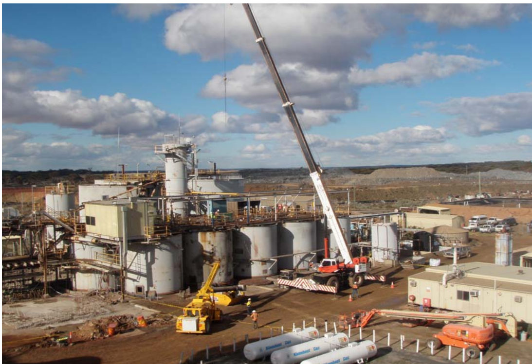
Figure 12: Refurbishment of CIL tanks and infrastructure
