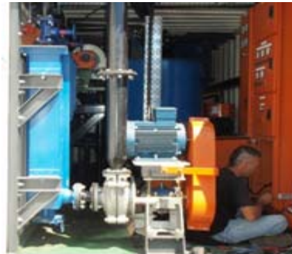
Venus Containerised Plant (above) Compact internal layout of Dense Medium Separation plant in container 2.
