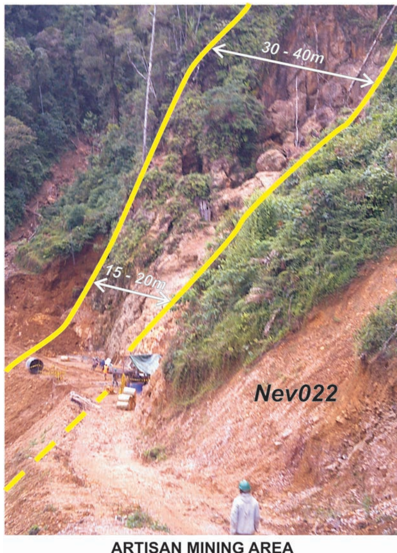
Figure 1: Drilling NEV022 at the Artisanal Mining Area
