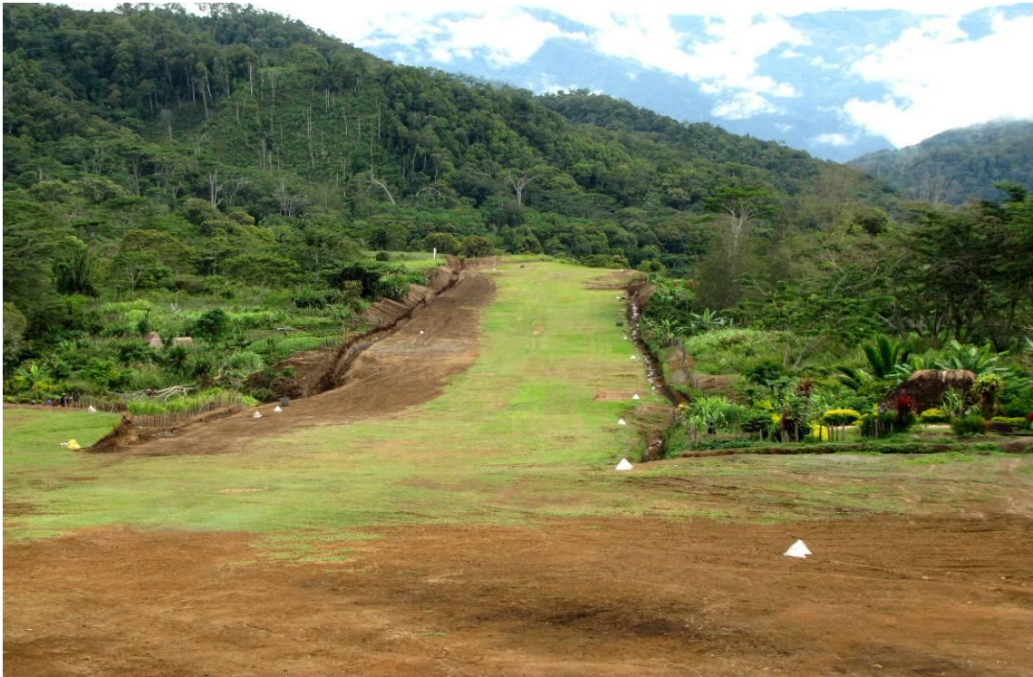
Upgrade of Gwasa airstrip including widening and digging drainage ditches
