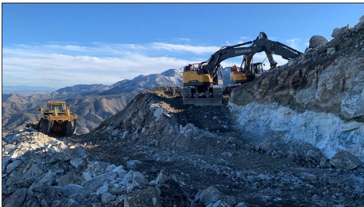
Figure 11 – Earthworks for two additional pads to improve access to southern Talon drill targets.
