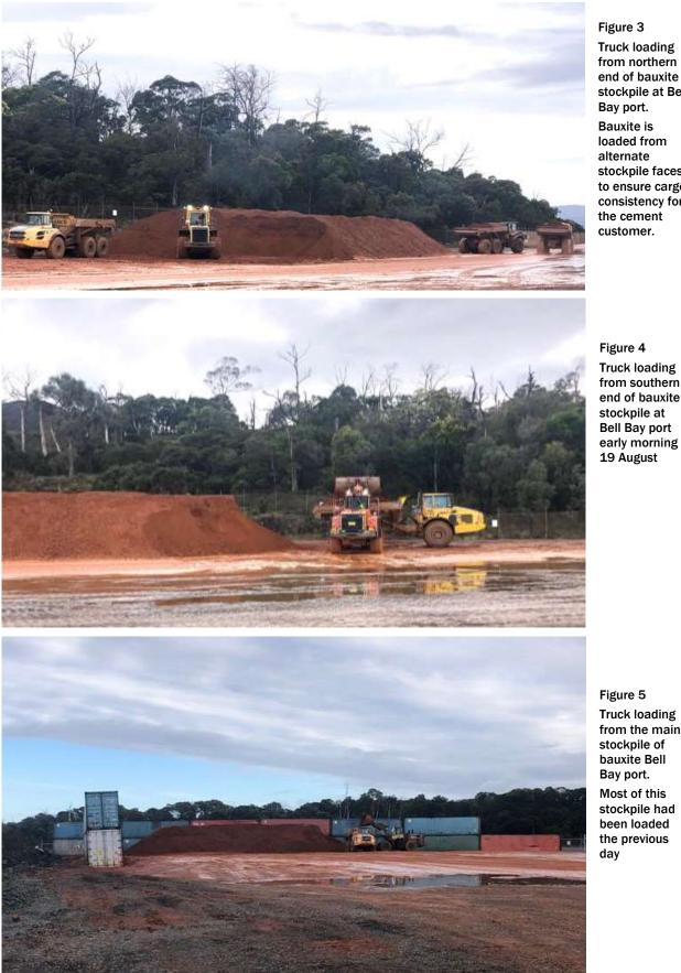
Figure 3 Truck loading from northern end of bauxite stockpile at Bell Bay port. Bauxite is loaded from alternate stockpile faces to ensure cargo consistency for the cement customer.
